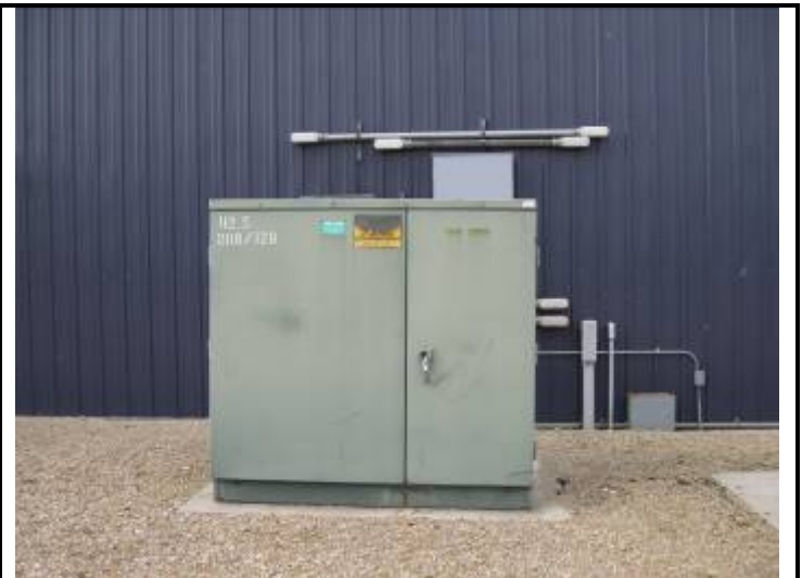
4. View of the pad mounted transformer located on the north side of the site building.
